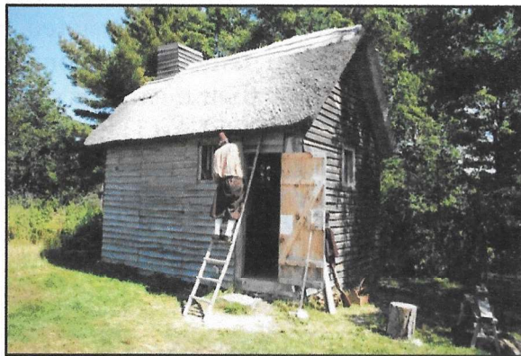
Reproduction of a 17th Century fisherman's home, typical of those found in New England, under construction.
